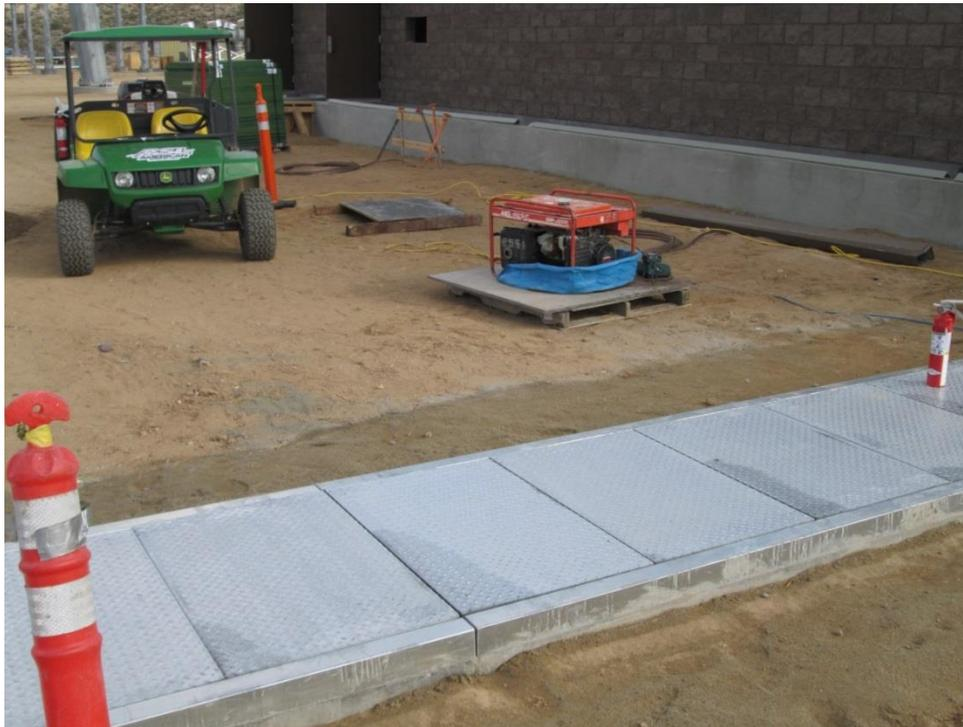
**Photo 8:** In accordance with MM-HAZ-1c, staged equipment, including generators, were equipped with drip pan containment to avoid hazardous materials leakage onto surrounding soil.
