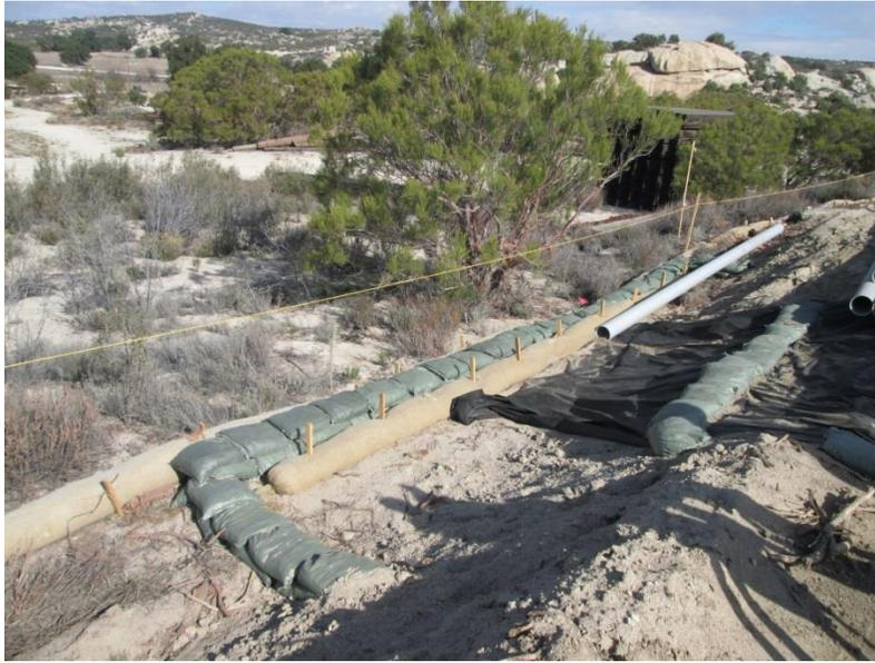
**Photo 3:** Erosion control devices such as straw wattles, gravel bag check dams, and silt fencing were installed along the project right of way in accordance with MM-HYD-1.
