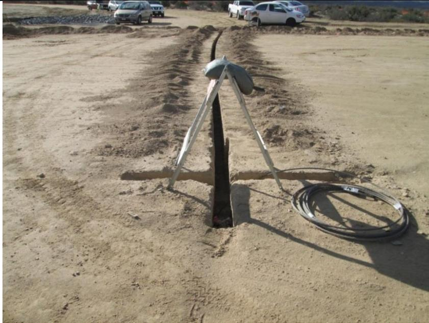
**Photo 7:** Biological monitors ensured all open trenches and excavations were either covered or left with an earthen ramp in accordance with MM-BIO-7a.
